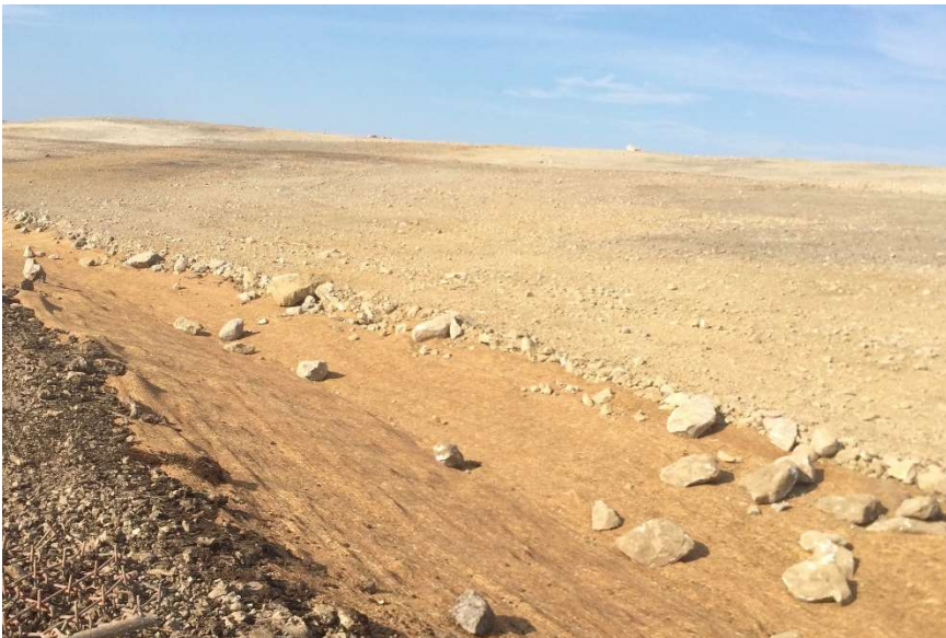
Erosion control blanket in channel. Note rocks pushed into channel to permit seeding of slopes.
