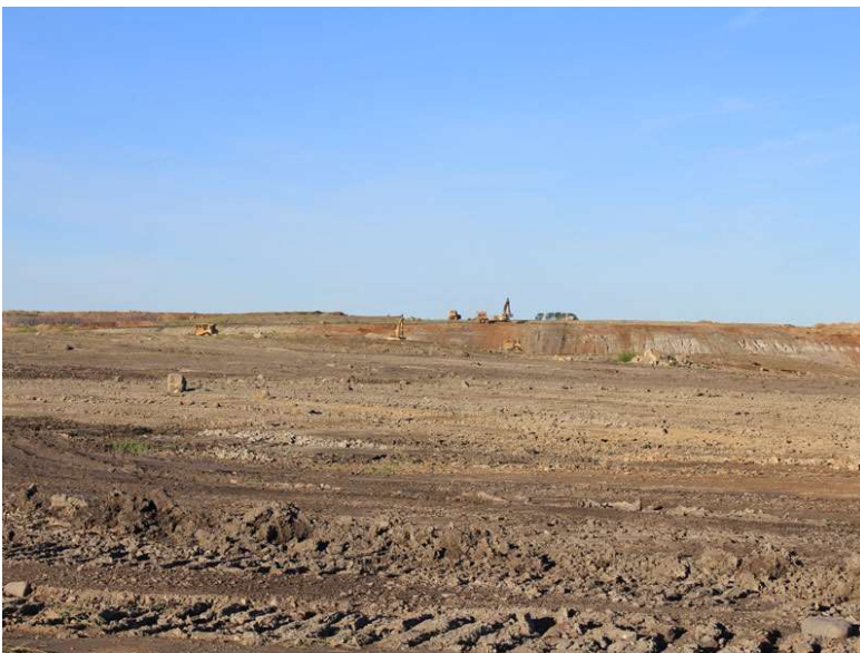
Typical conditions prior to seeding. Soils include a range of waste rock, clay and till but contain no organic content. The soils are generally non acidic and were directly revegetated.
