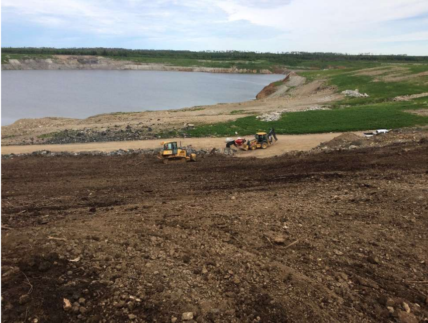
Seeding of future shorelines in flooded open pits on 3:1 slopes. As opposed to waste pile seeding the design did include a light amendment of topsoil.
