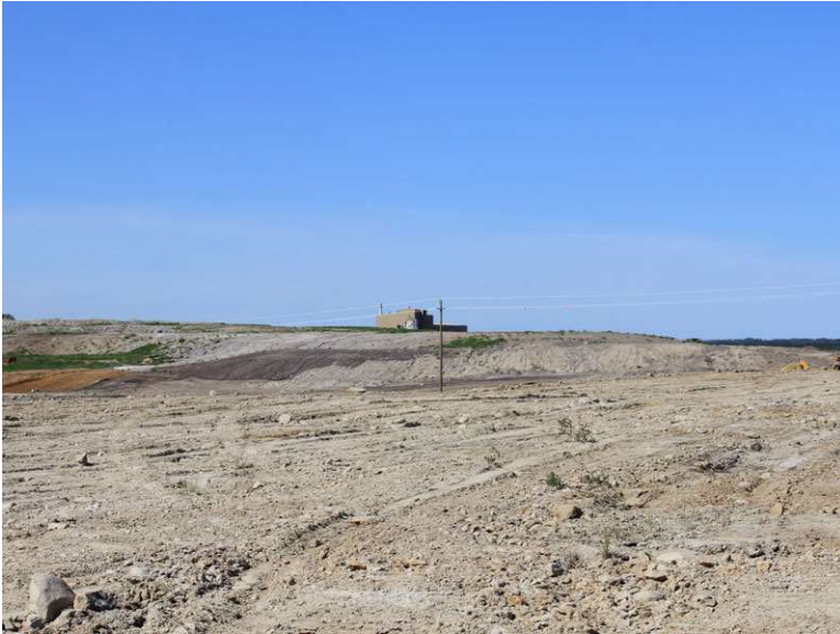
Waste rock clay and till following rough grading by earthworks contractor.
